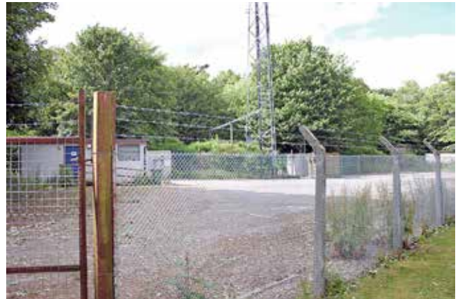
Exterior view of site. The 1980s portacabin can be seen to the left of the image. This was the main base for staff stationed here until 2016
